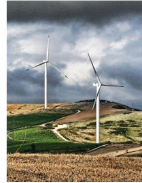
Wind farm monitoring in Portugal
