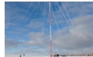
Site Assessment in Cold Climate
